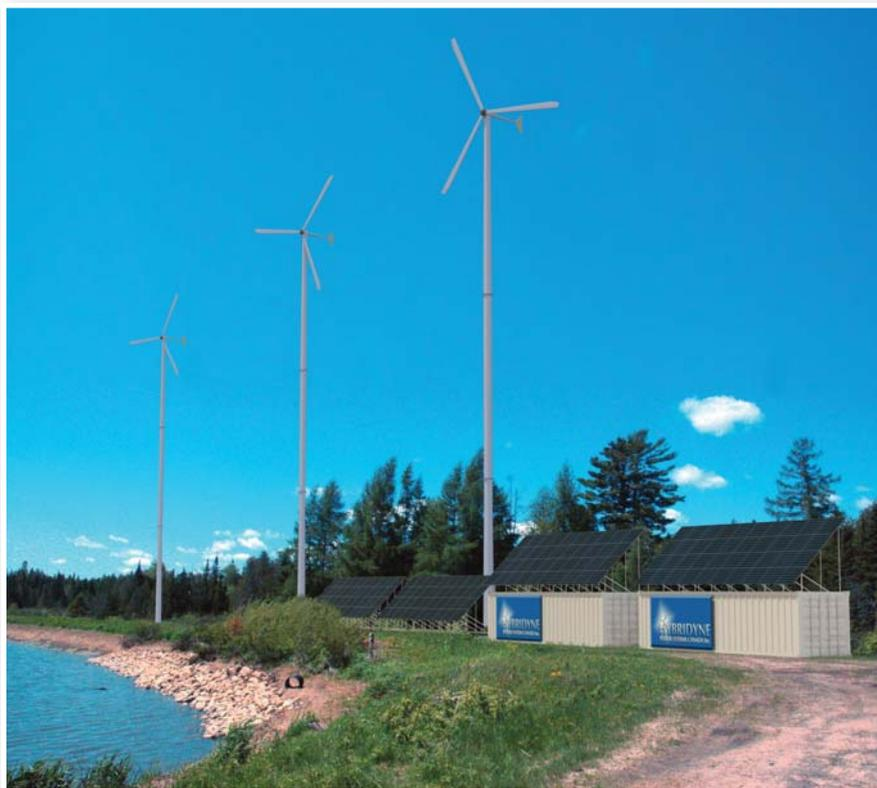
*Hybridyne's proposed system consisted of twelve 10-kW wind turbines and 48 kW of photovoltaic solar panels.*
